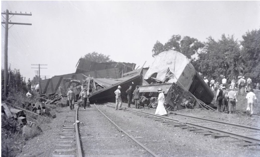
A steam powered crane in the ditch. Ohio Memory Collection
